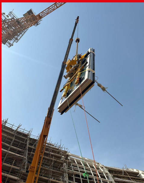
PREFABRICATED ELEMENTS FOR THE OMAN
